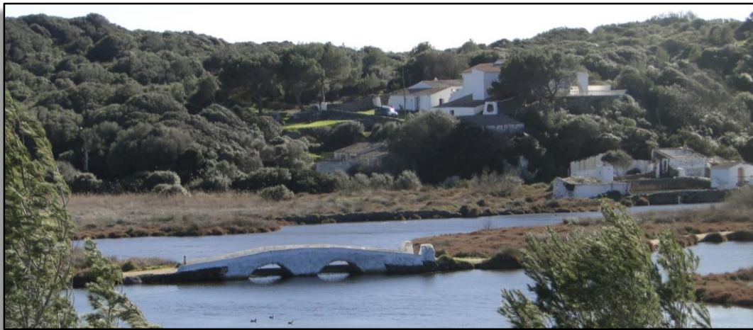
Bridge with the floodgates used to control the flow of water between S'Albufera and the sea. This form of control was traditionally used for fishing purposes, but today it is geared towards conservation of the lagoon.
